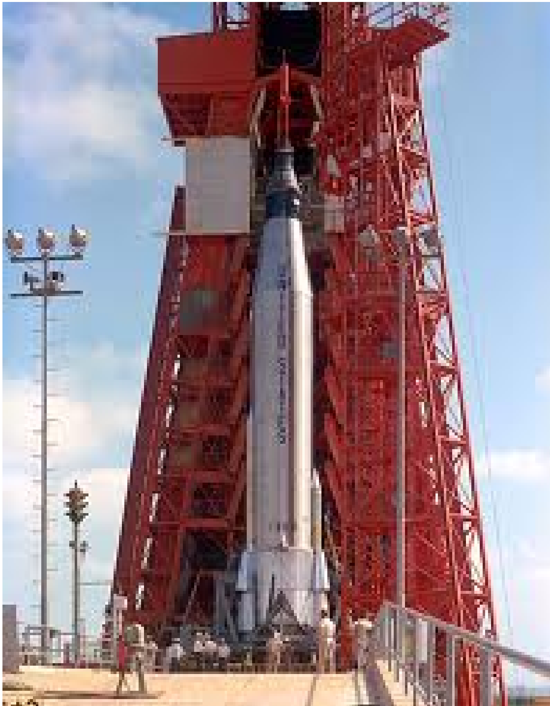
Figure 5: Atlas Missile Test Stand Service Tower
